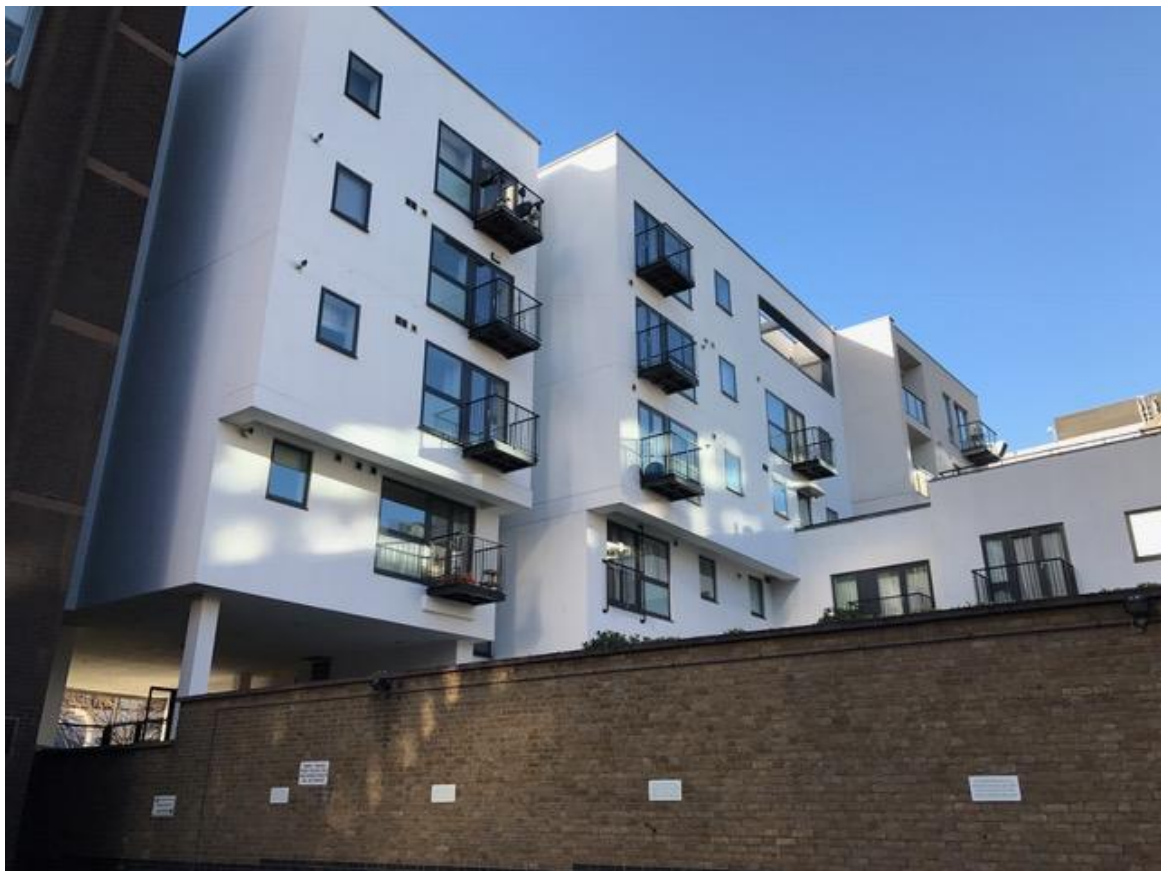
Image 1 – View from the site towards Thackery Court and Dickens Mews
